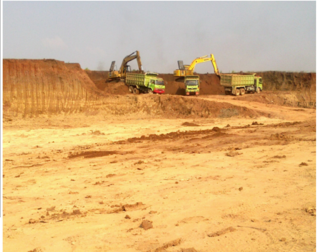
Cut and Fill Work in Phase 3
