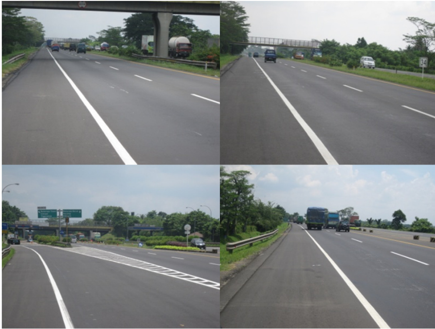
Improvement on Tangerang-Merak Toll Road
