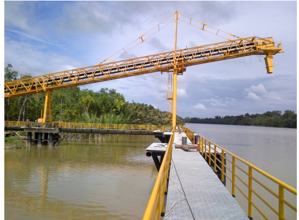
Construction of Jetty, East Kalimantan
